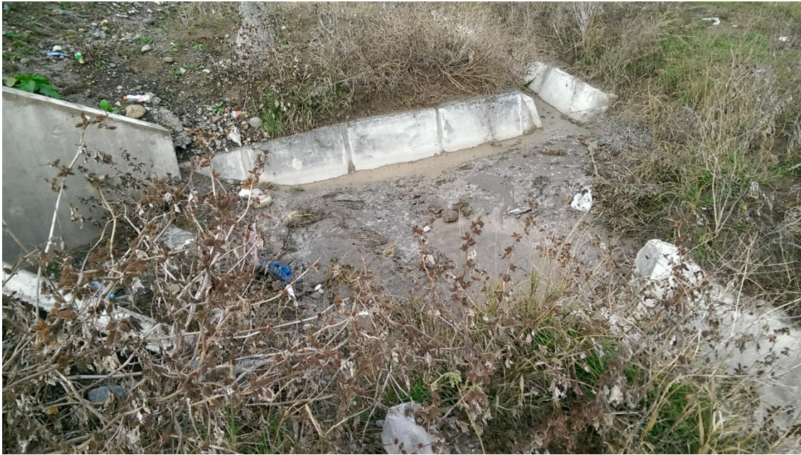
Picture 3. Dismantling of the existing concrete culverts
