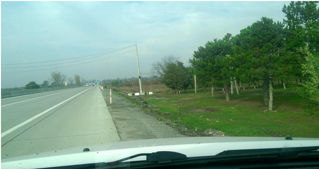
Picture 1. Existing high voltage power line
