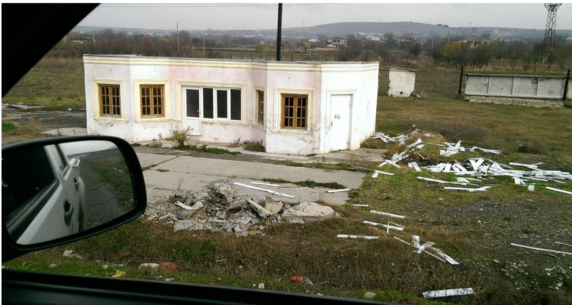
Picture 4. Structure to be demolished
