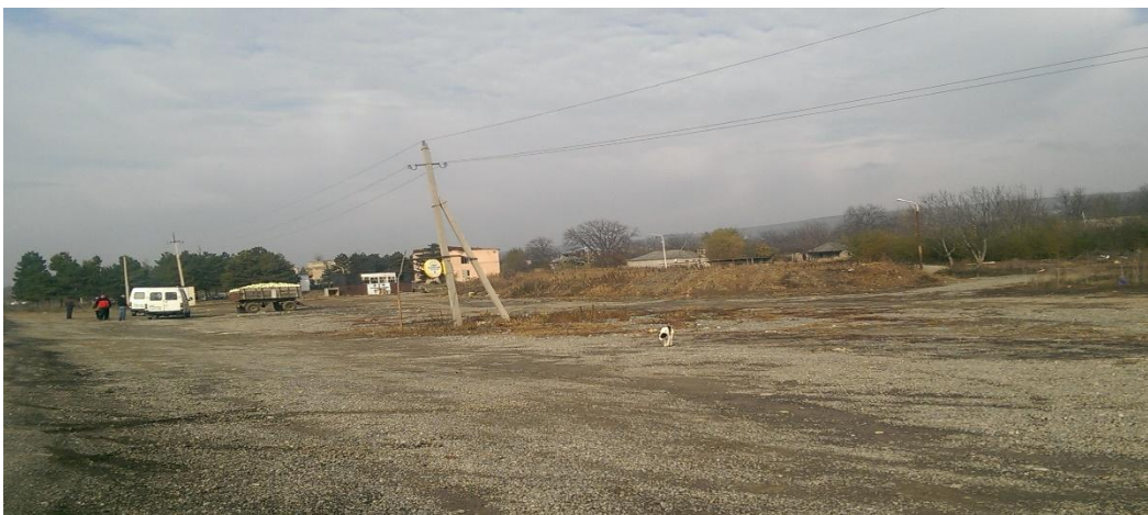
Picture 2. Existing high voltage power line
